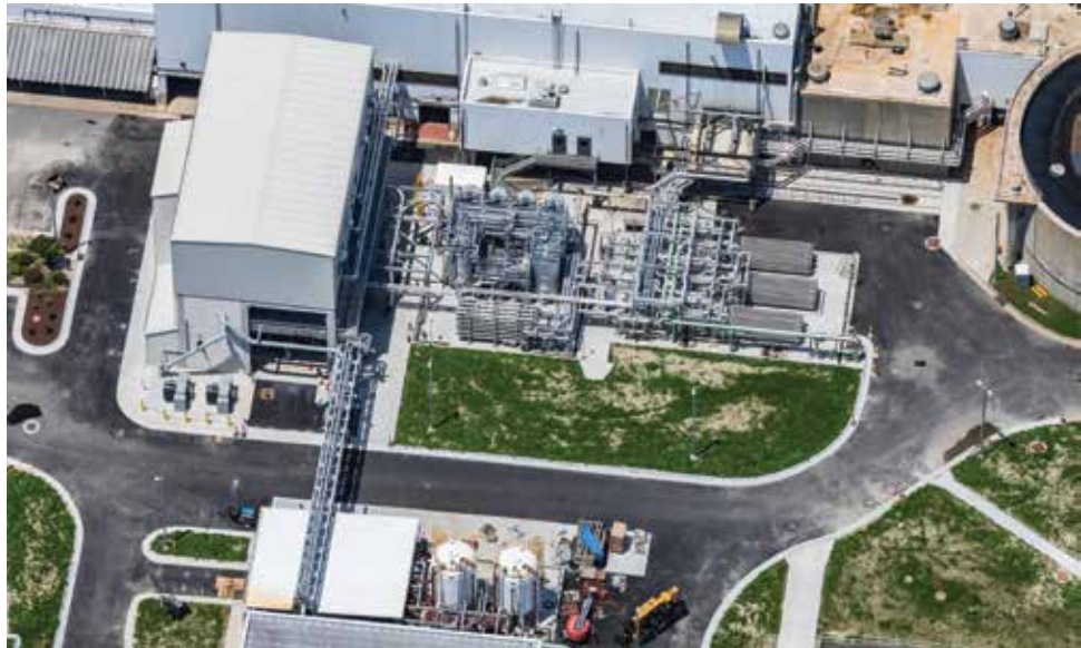
The Cambi thermal hydrolysis process (THP) system allows the Hampton Roads Sanitation District (HRSD) in Virginia to generate power and fine fertilizer directly from sewage waste.
